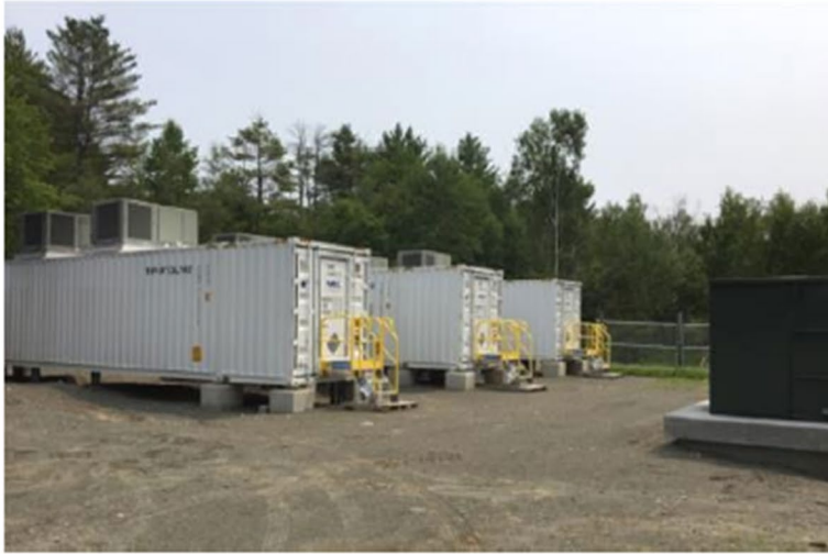
Shipping units containing 950 lithium-ion batteries in Madison, Maine. This project has a capacity of just under 5 MW that can help supply power and balance electricity demand daily. Image Source: New England Battery Storage
