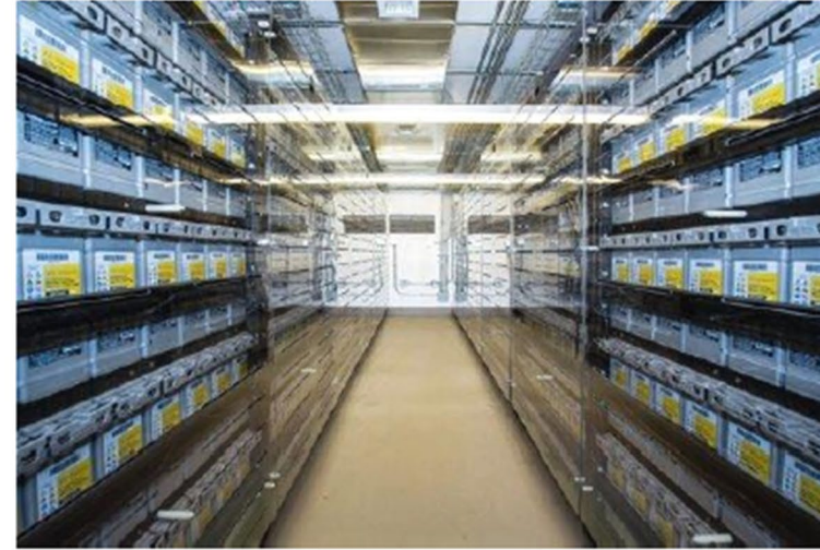
Batteries stacked inside of a shipping container in Boothbay, Maine. Image Source: Convergent Energy
